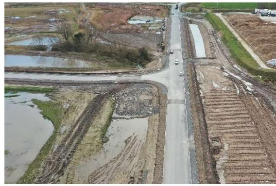
**Image 04:** Showing Topsoil works complete ready to receive seed
