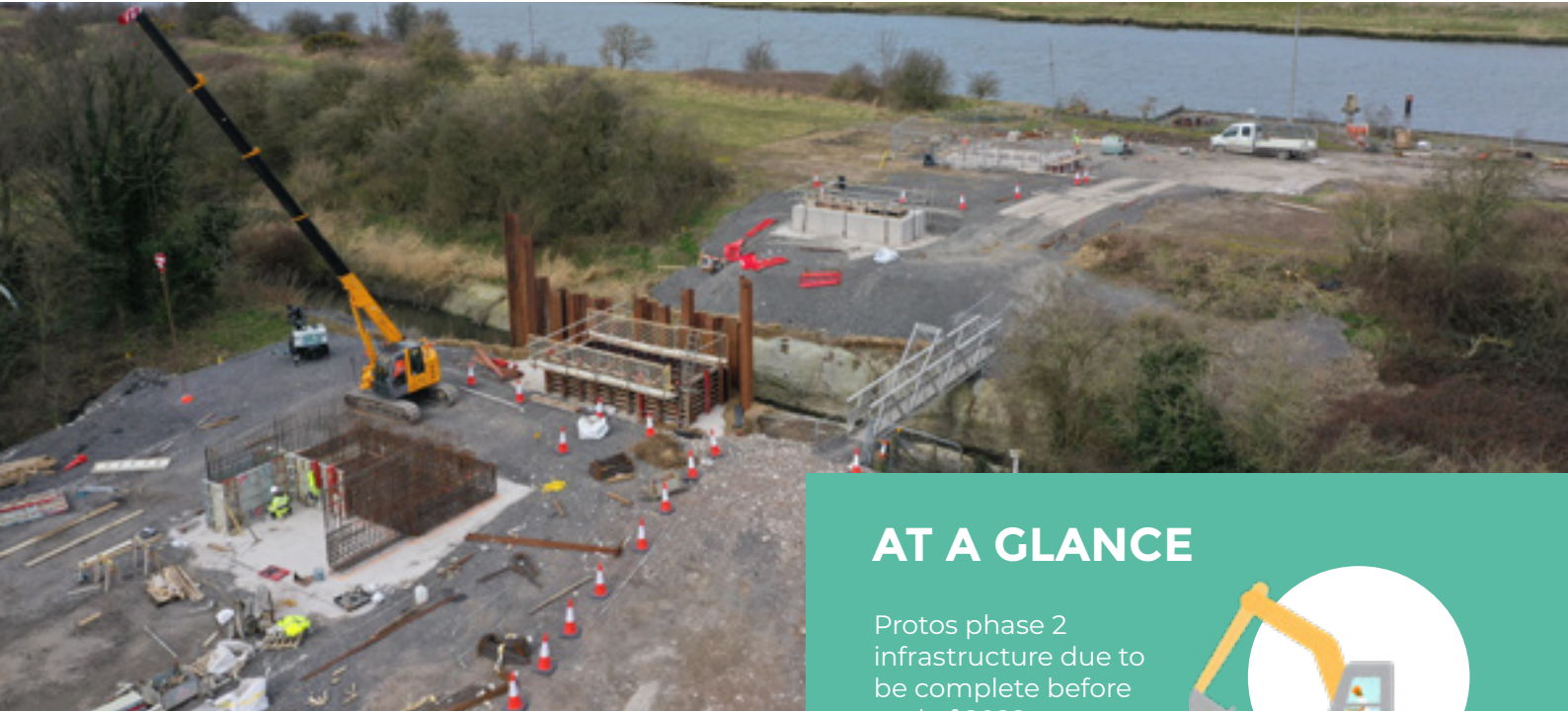
Construction of Tang Bridge as part of the Phase 2 Infrastructure Works.
