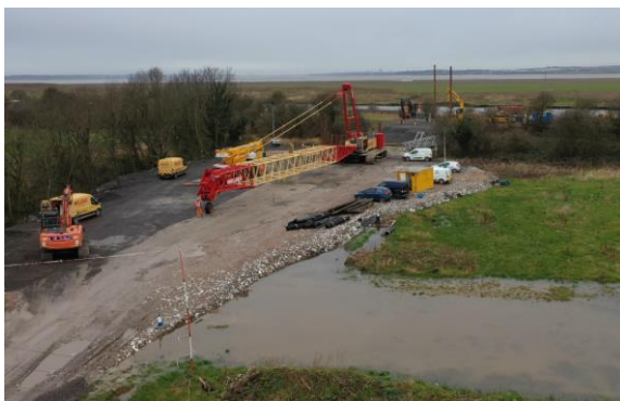
Image 03: Showing TANG Bridge Construction
