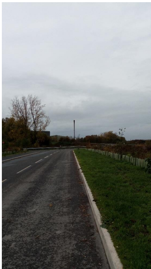
Figure 3. Access road serving the site
